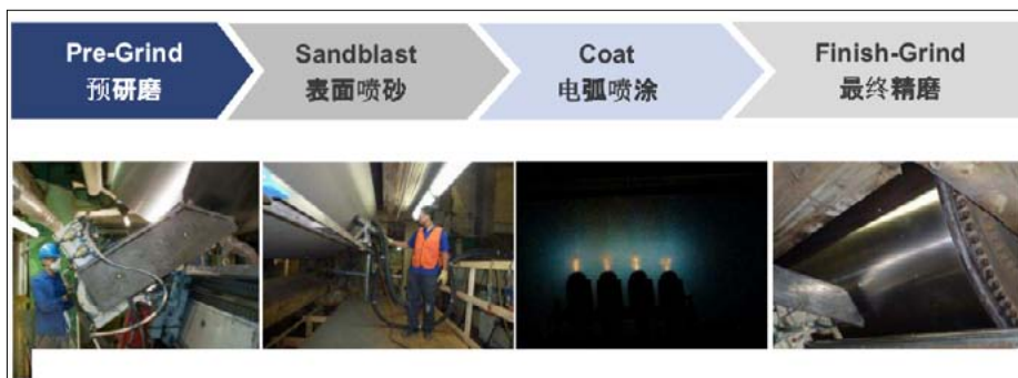
Figure 3 The Specific Process of Steel Yankee Dryer Spraying
