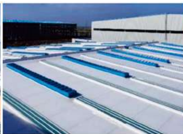
铺设TPO防水卷材
